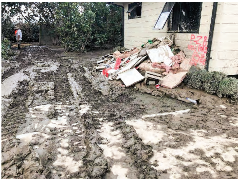
A house in Pakowhai, Hawkes Bay in the aftermath of Cyclone Gabrielle.
